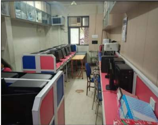
Air Conditioners Installed in Lab
