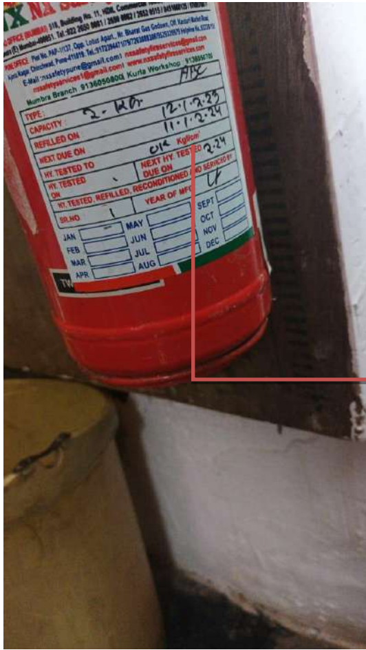
Fire extinguisher is updates.
