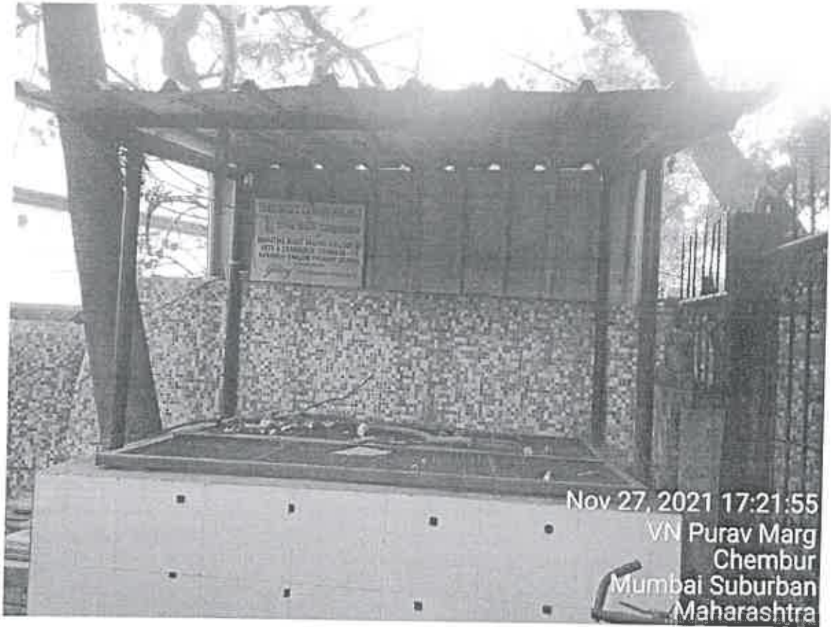
Solid Waste Management- Compost Pit
